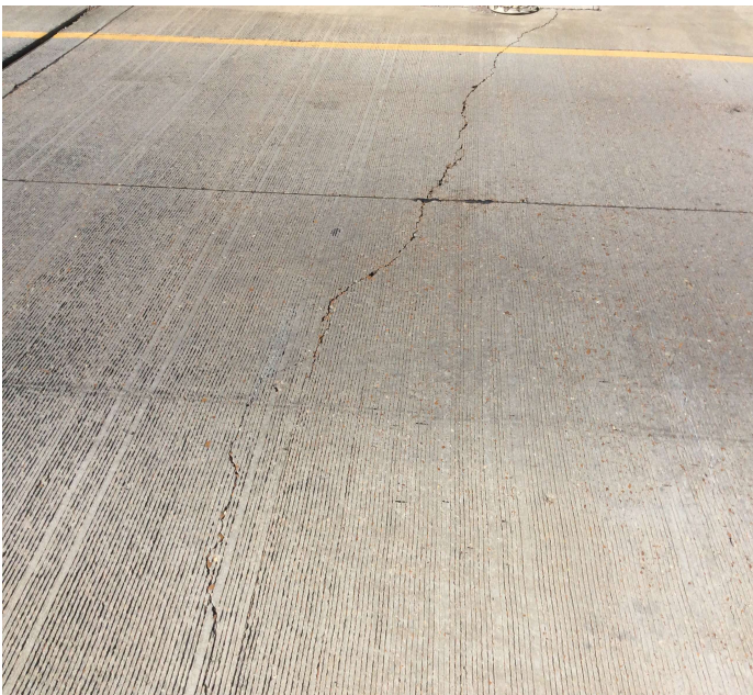
PHOTO 1 Description Typical approach slab cracking.
