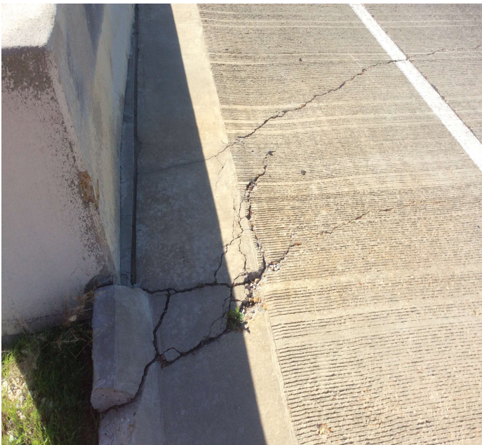
PHOTO 1 Description Typical approach gutter cracking.
